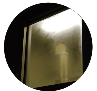
A lead glass surface fogged because its surfaces was leaved wet condition.
